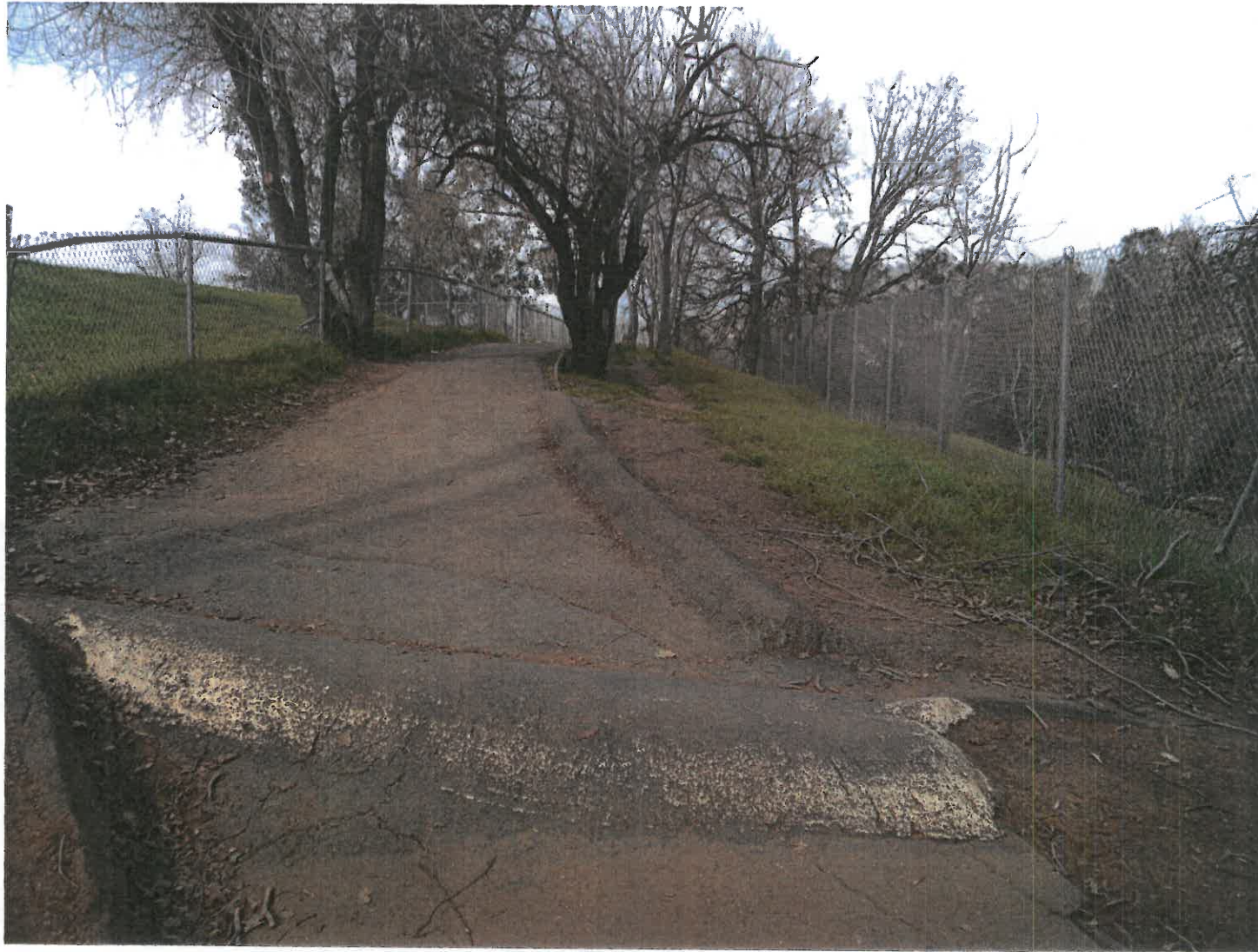
(#12) Drainage berm at the uphill side of trail.
