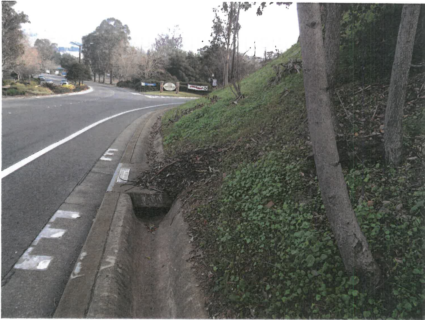
(#20) Catch basin at the bottom of the hill.
