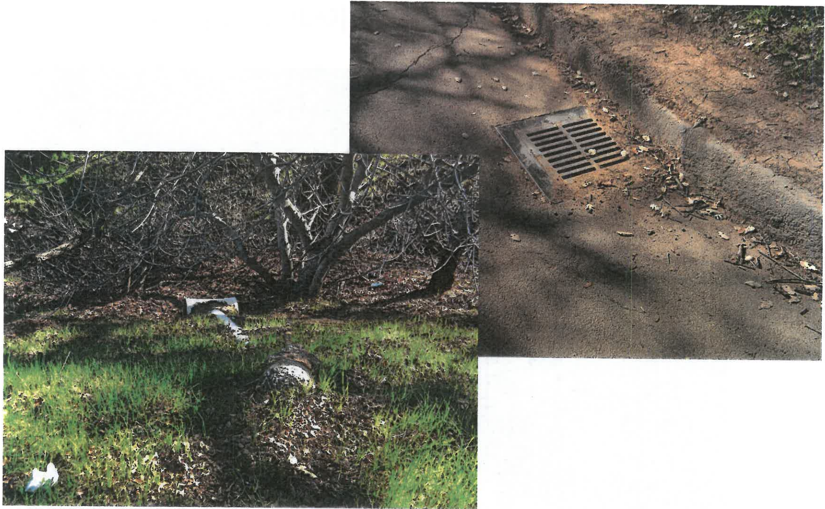
(#17) Typical drain inlet along the trail piped out the hill.
