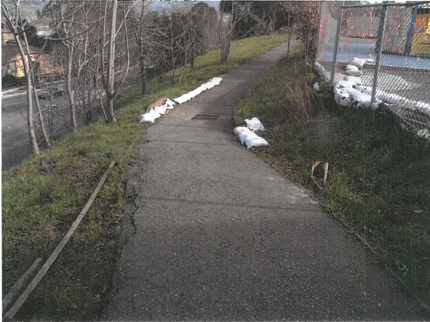
(#24) Asphalt curb to replace wood backing and sandbags.
