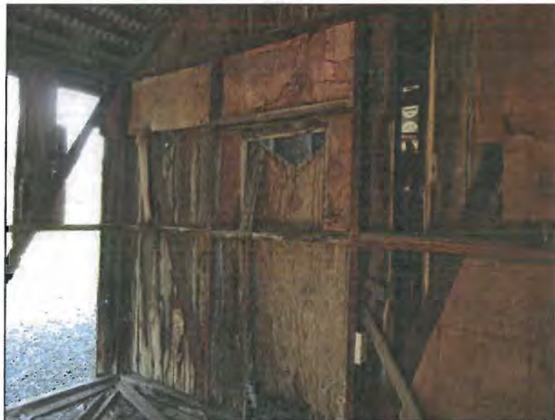
Figure 5. Photograph of the work shed outbuilding interior taken during field visit in November, 2015.
