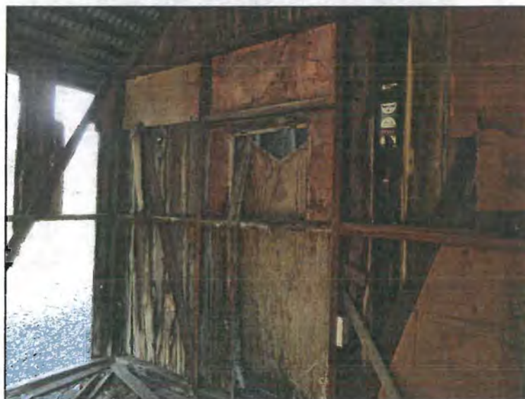
Photograph of work shed outbuilding interior, taken during field visit in November, 2015.
