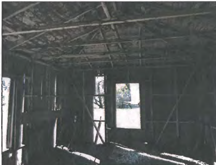
Photograph of garage outbuilding interior, taken during field visit in November, 2015.
