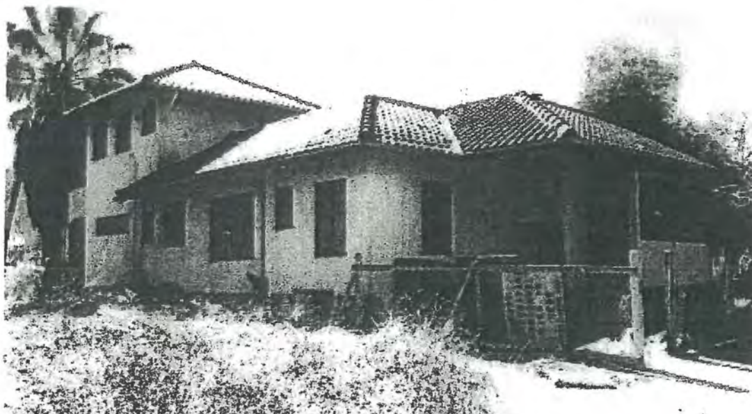
East & north facades, facing south, 2001
