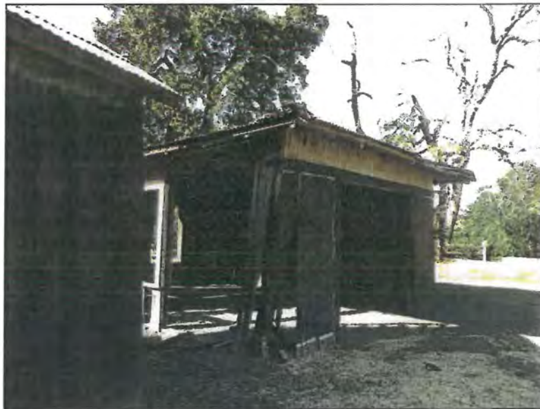
Figure 11. Photograph of the garage taken in 2015 by ECORP
