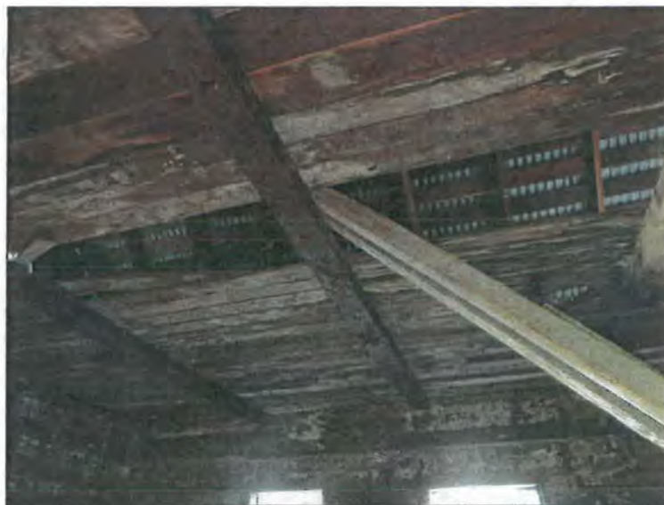
Photograph of granary outbuilding interior, taken during field visit in November, 2015.
