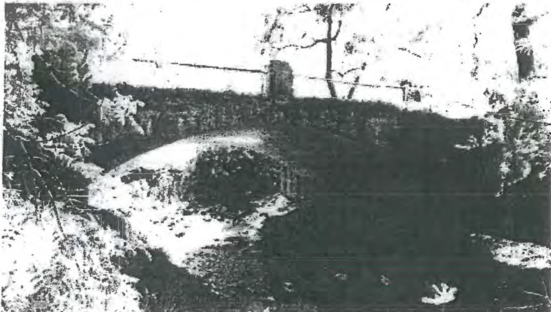
Keller Bridge, facing southeast, 2001
