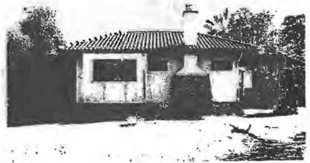
West Facade, 2001, kitchen and screened porch behind trees at left
