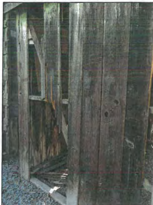
Photograph of work shed outbuilding exterior, taken during field visit in November, 2015.
