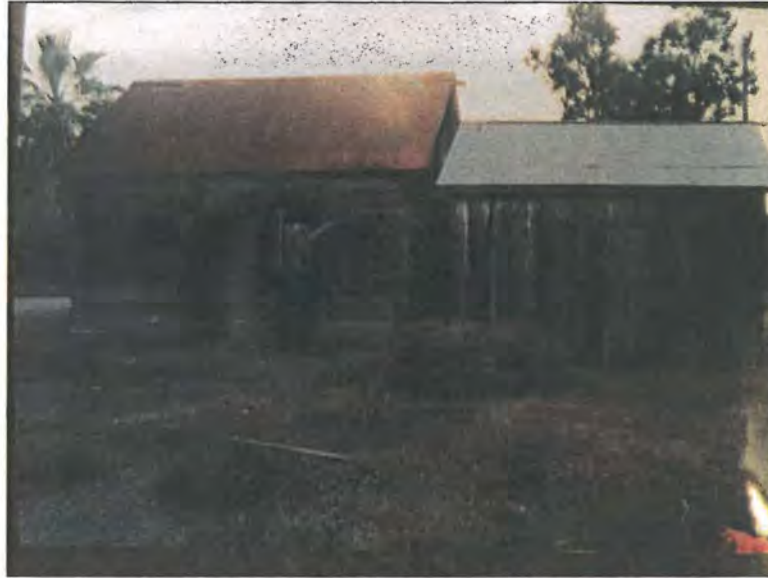
Photograph of the granary and work shed taken in 2001 by Saxby
