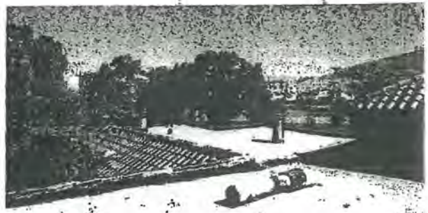
Roof looking north, 2001
