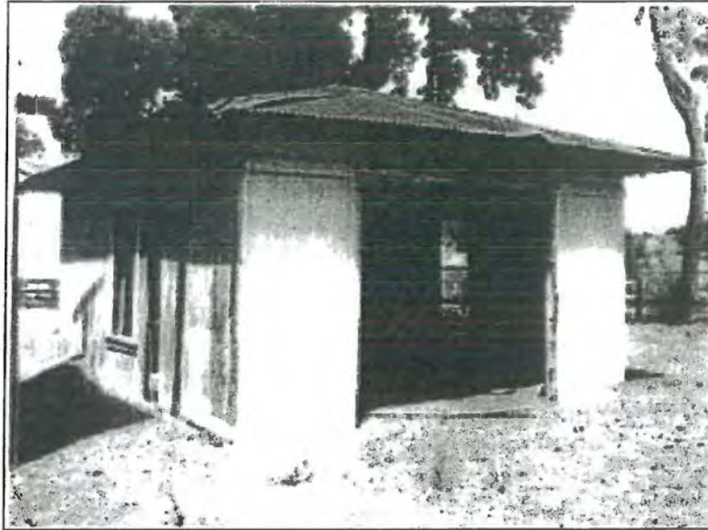
Figure 10. Scanned image of a photograph of the garage taken in 2001 by Saxby
