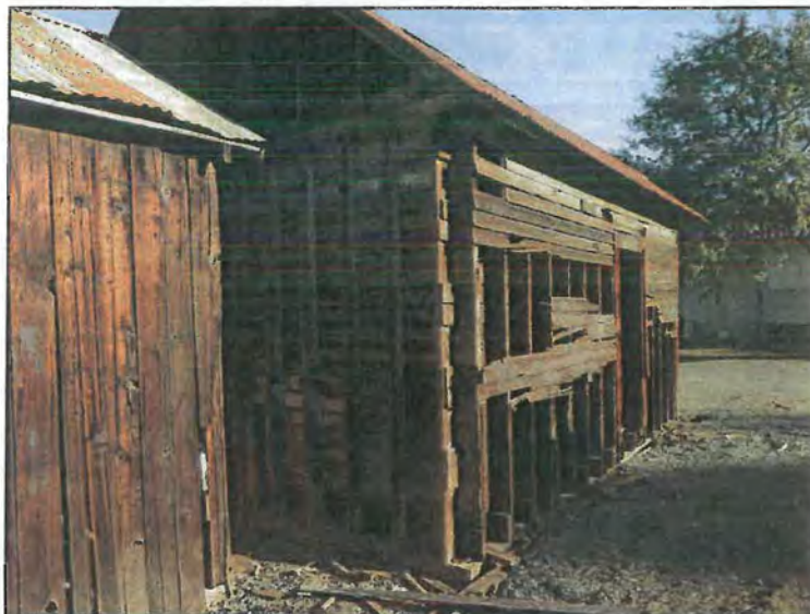
Photograph of granary outbuilding exterior (western facing wall), taken during field visit in November, 2015.
