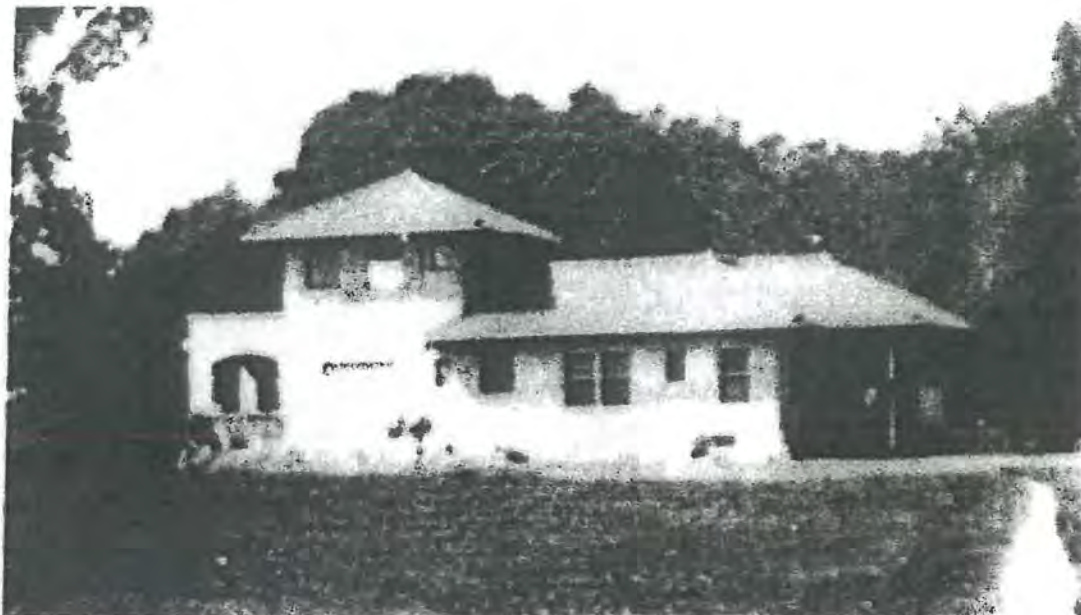
East facade, facing southwest, ca. 1920's
