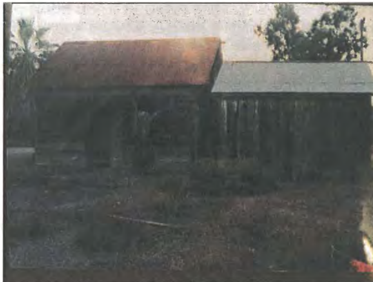
Figure 8. Photograph of the granary and work shed taken in 2001 by Saxby
