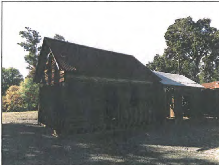
Photograph of the granary and work shed taken in November, 2015 by ECORP
