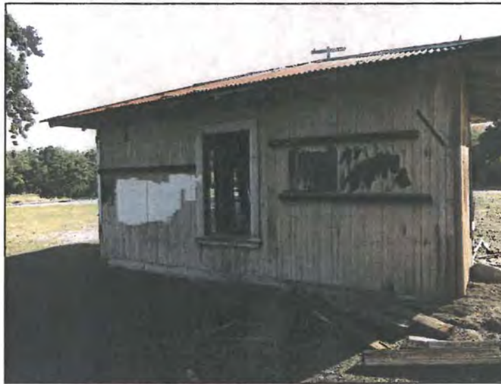
Photograph of garage outbuilding exterior (northern facing wall), taken during field visit in November, 2015.
