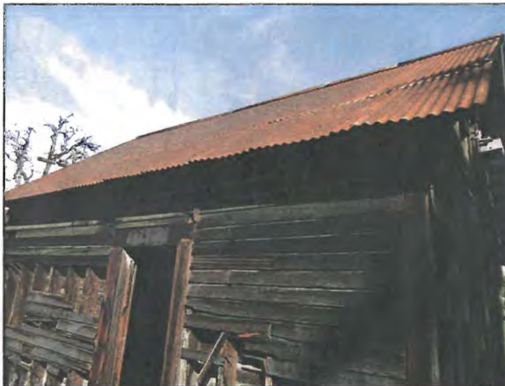
Photograph of granary outbuilding exterior, taken during field visit in November, 2015.
