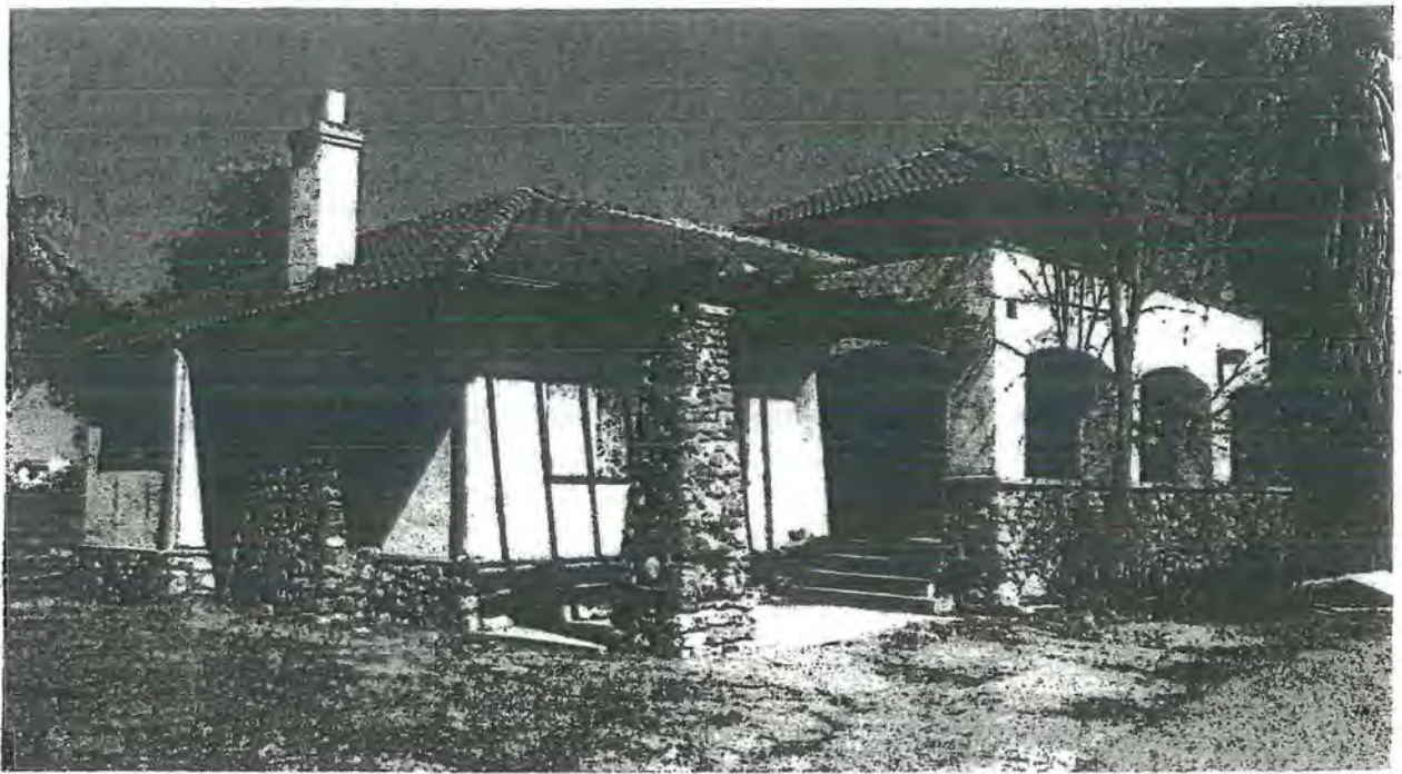
Keller House, west & south facades, 2001
