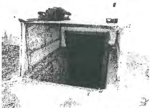
Cellar access, facing south, 2001
