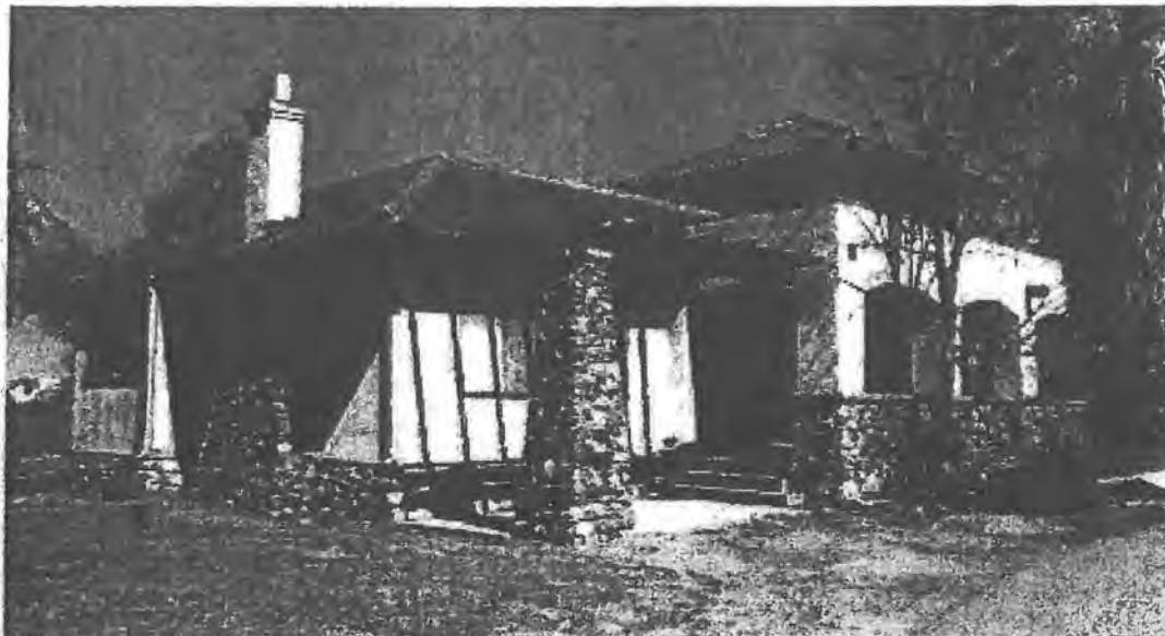
Keller House, west & south facades, 2001
