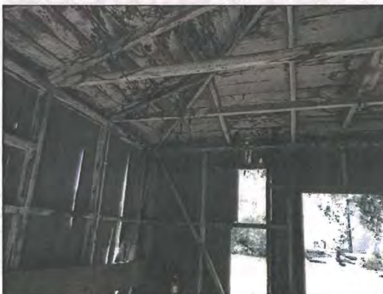
Figure 7. Photograph of the garage outbuilding interior taken during field visit in November, 2015.
