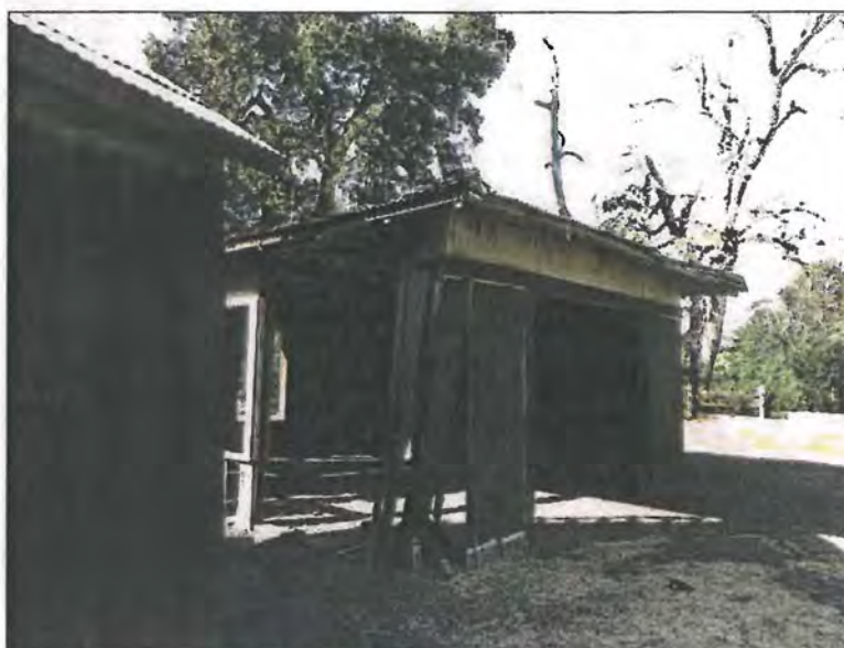
Figure 6. Photograph of the garage outbuilding exterior taken during field visit in November, 2015.
