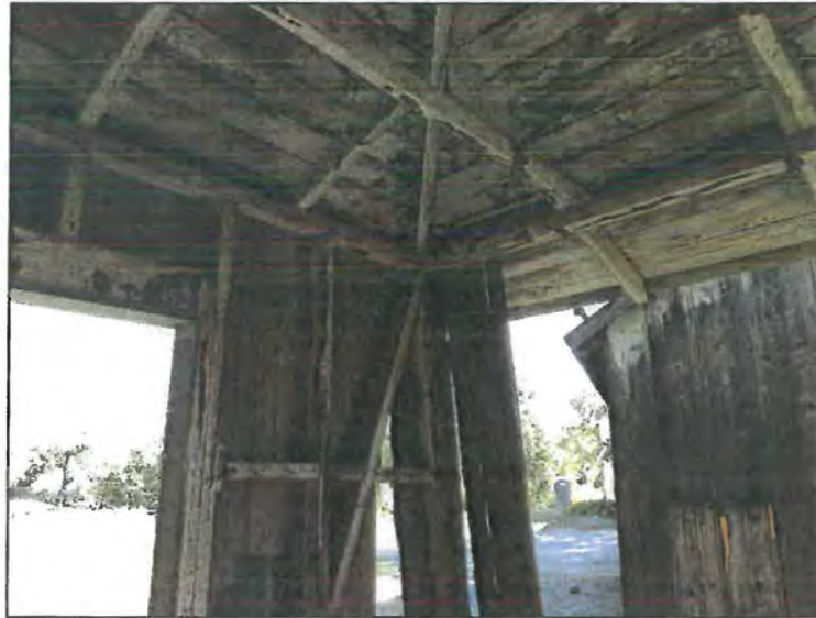
Photograph of garage outbuilding interior, taken during field visit in November, 2015.
