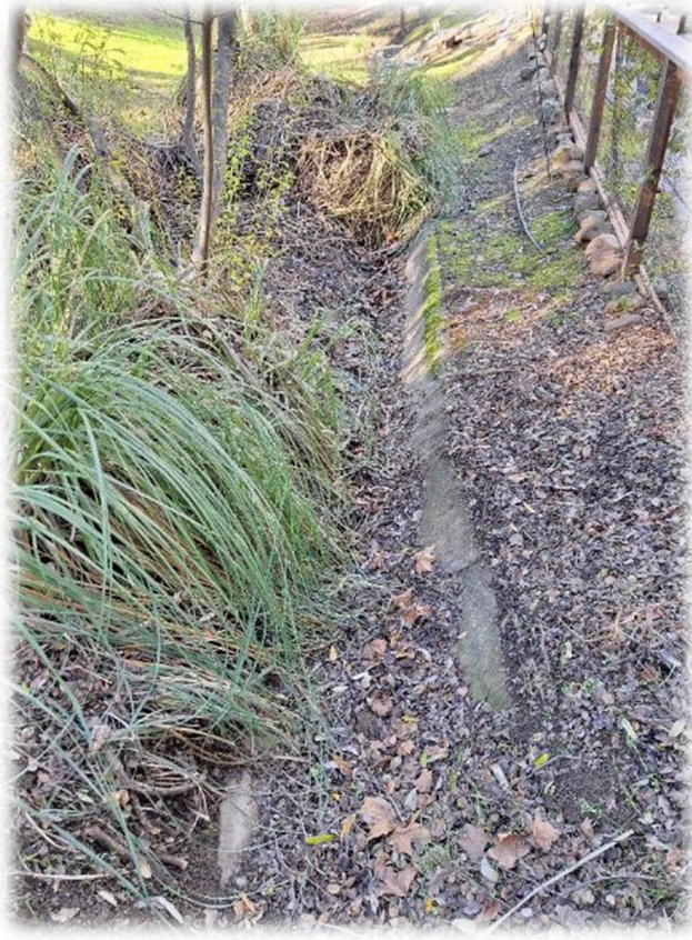
Photograph 6 – V-ditch at 321 Windmill Canyon Place. All remaining V-ditches and drop inlets in the area should be checked and cleaned.
