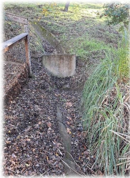
Photograph 5 – Drop inlet and V-ditch require cleaning at 321 Windmill Canyon Place.
