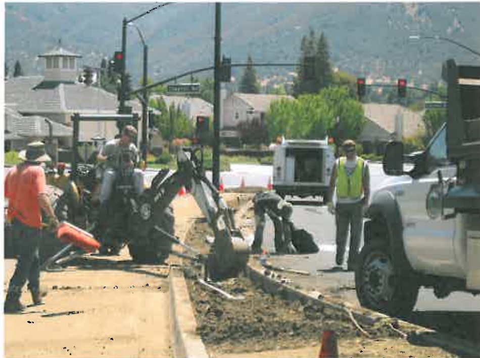
City Maintenance Staff and Seasonal Workers preparation of Oakhurst Median Noses for decorative hardscape treatment July 30 2010
